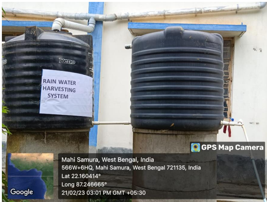
Figure 6: Geo-tagged photographs of roof-top rainwater harvesting system installed at Government General Degree College, Keshiary purposed for watering of the college garden and aquaculture unit
