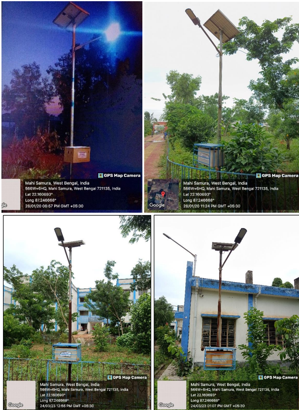
Figure 1: Geo-tagged photographs of solar powered lamp posts installed at Government General Degree College, Keshiary to tap alternate source of energy for illumination of the campus during the dark hours.
