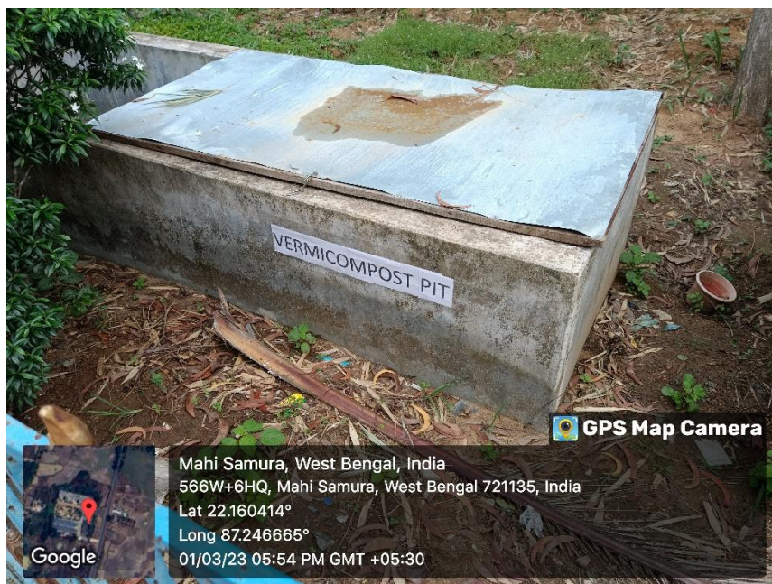
Figure 2: Geo-tagged photographs of a construction pit within the college campus repurposed for vermicomposting for processing biodegradable wastes
